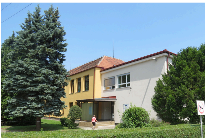
School After the Refurbishment
