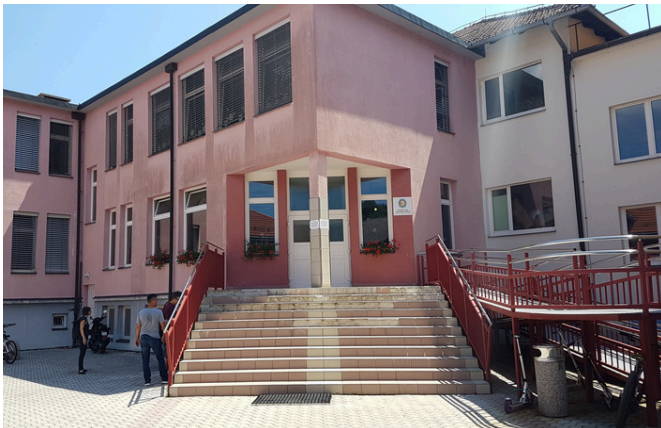
School Before the Refurbishment
