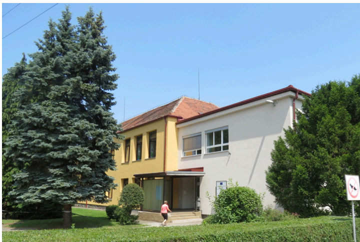
School After the Refurbishment
