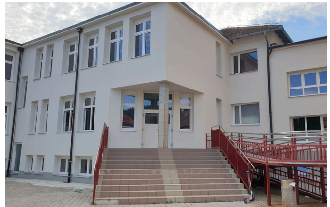
School After the Refurbishment
